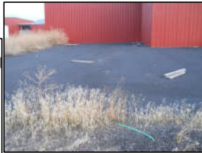
Asphalt Cap over soil contamination in Prineville
